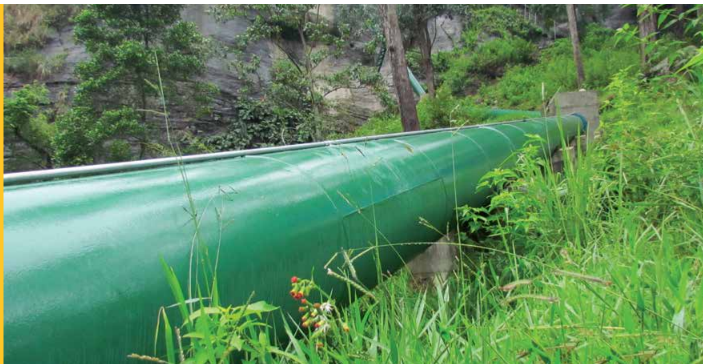
LAUGFS Power pipeline in Balangoda
