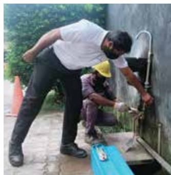
Foot operated washbasins made of damaged cylinders.
